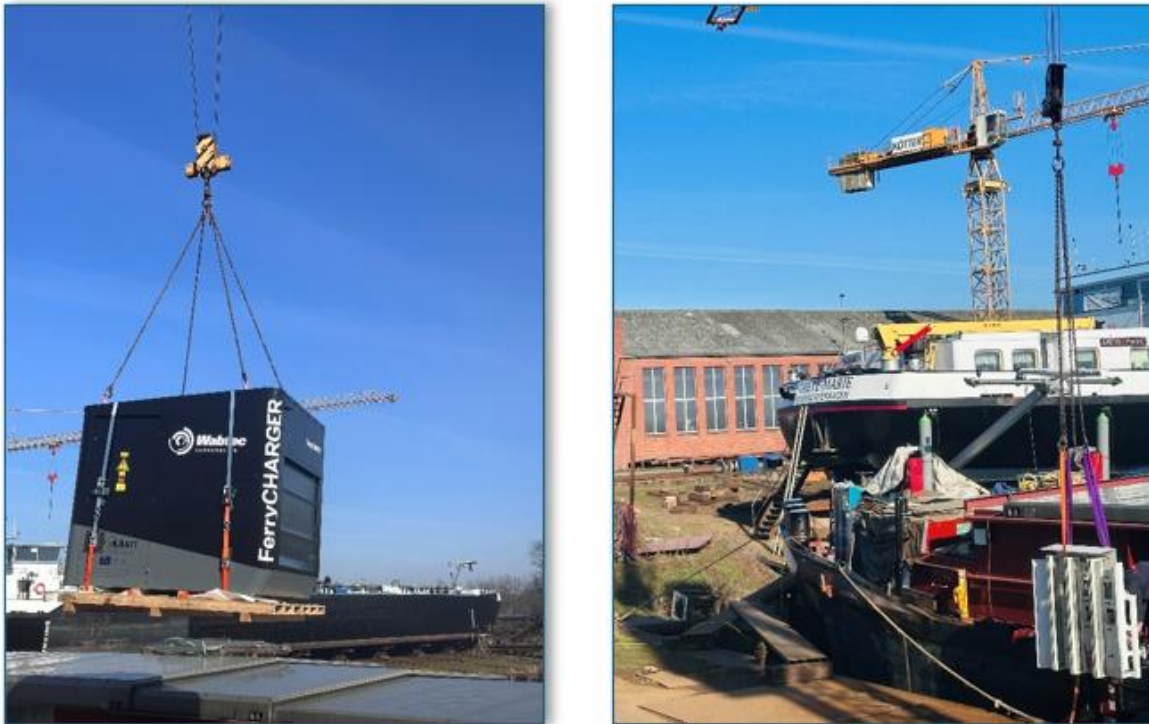
Figure 5 Installation of EVSE 1 connection system for EV 2
