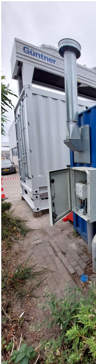
Figure 5 assembled combination of baseframe, multi-MW charger container and dry cooler on top viewpoint: left image: left side: MV switchgear doors, right side: AC connection for testing. Right image: left side: bottom grid-iron for transformer air-intake, right side: AFE1 power conversion and protection compartment doors.
