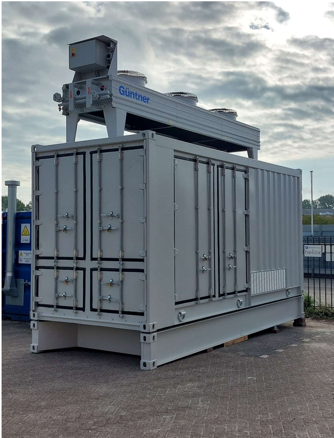
Figure 4 assembled combination of baseframe, multi-MW charger container and dry cooler on top viewpoint: left; LV DC output side with cable connections behind bottom doors, right; AFE2 power conversion and protection compartment doors, far-right: bottom grid-iron for transformer air-intake.
