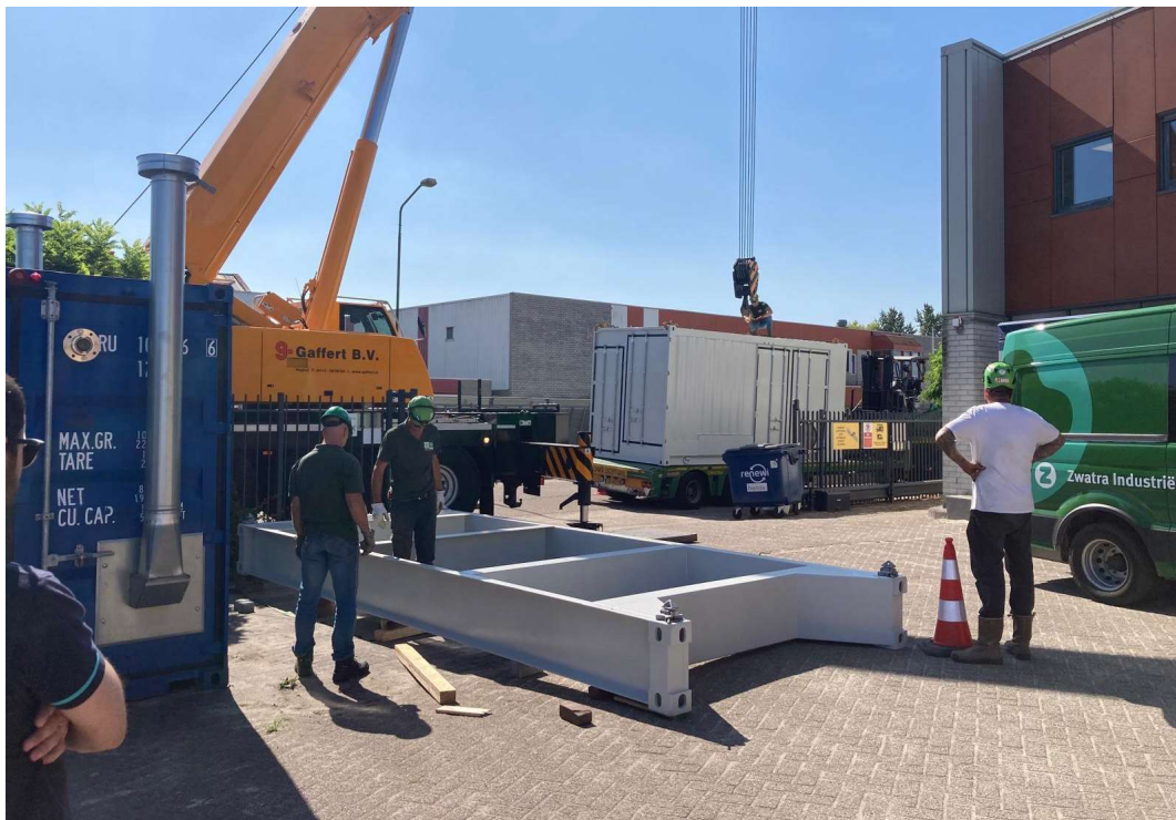
Figure 1 placement of baseframe at testing site
