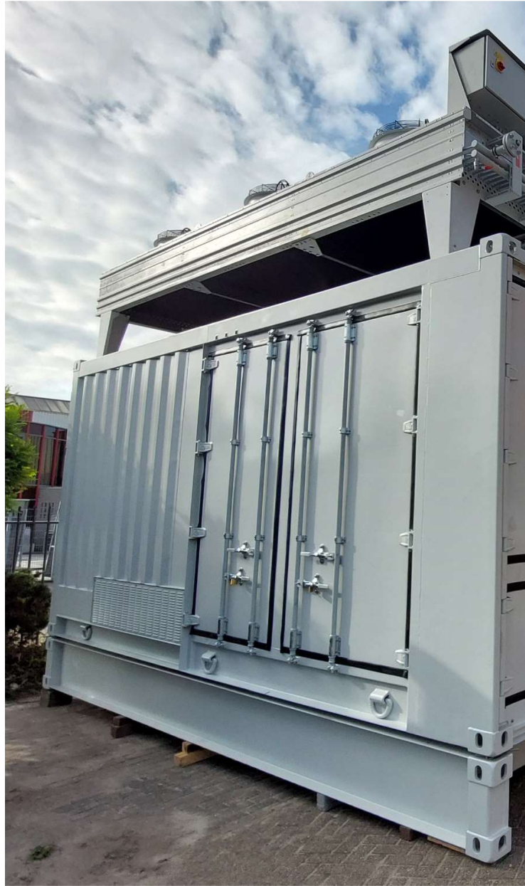
Figure 5 assembled combination of baseframe, multi-MW charger container and dry cooler on top viewpoint: left image: left side: MV switchgear doors, right side: AC connection for testing. Right image: left side: bottom grid-iron for transformer air-intake, right side: AFE1 power conversion and protection compartment doors.
