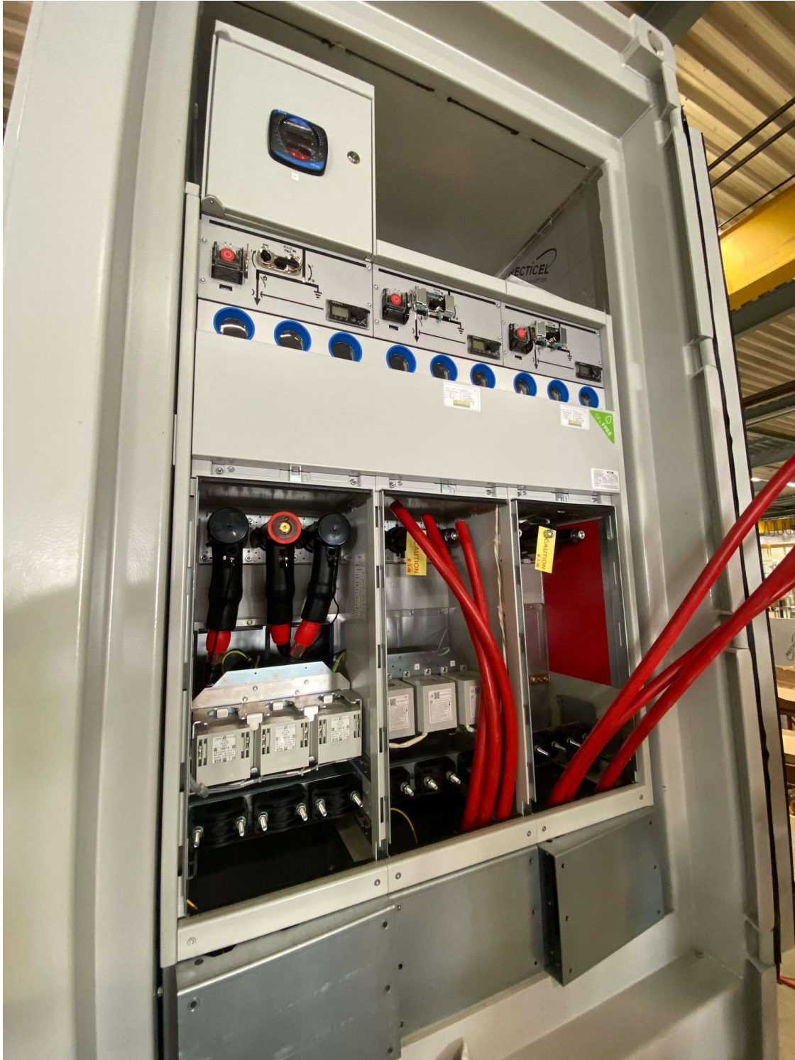
Figure 7 Mounted MV switchgear set and MV cables installation
