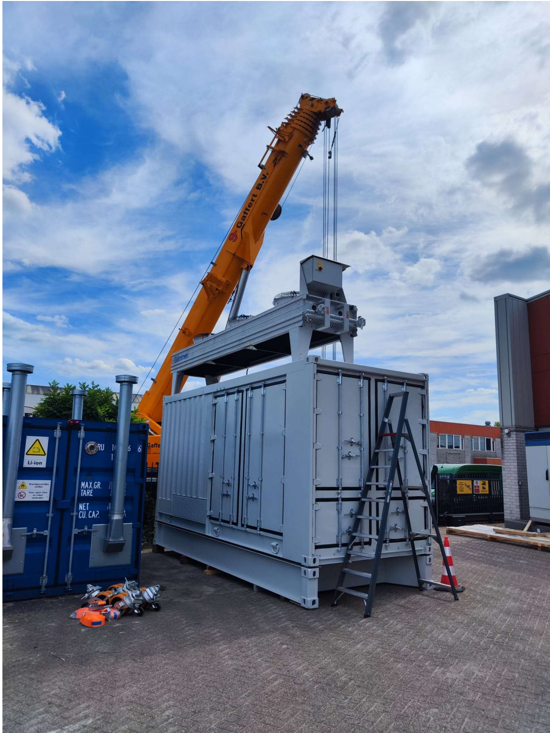
Figure 3 placement of the dry cooler on top of the baseframe and multi-MW charger
