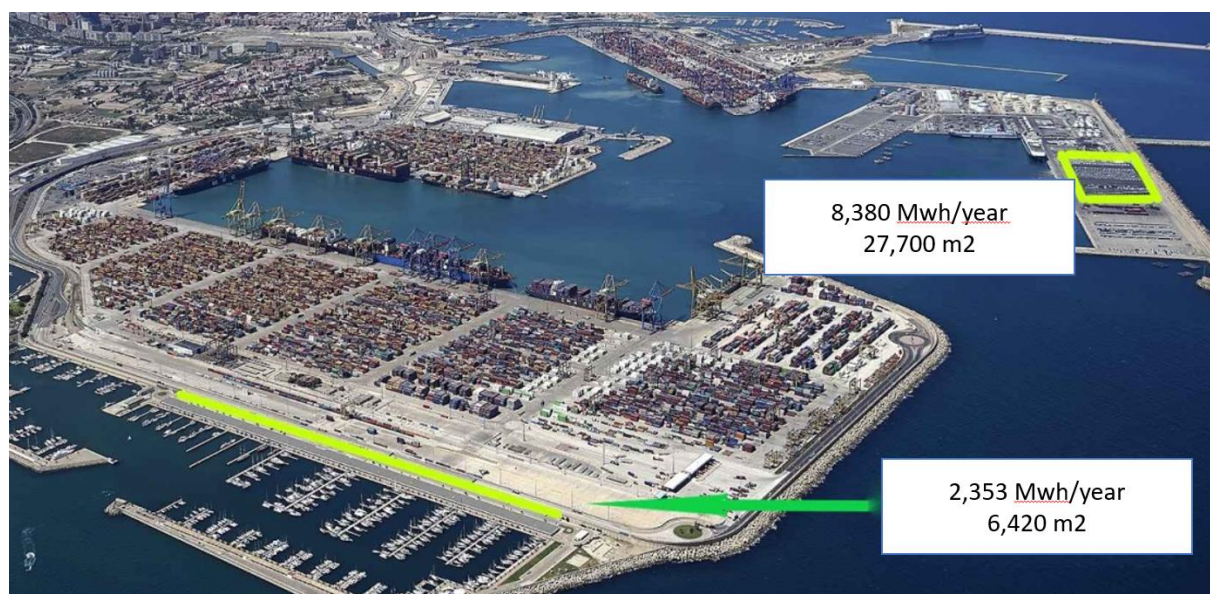
Figure 8 : Valencia port overview with the future PV plant installation area
