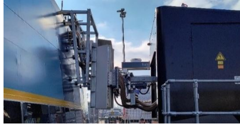
Figure 9 Same ship (dual) connection mated with manual connection (left) and temporary HYPOBATT ACD connection (right)
