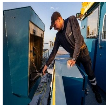
Figure 10 Manually operated dual-MCS plugging into the vessel
