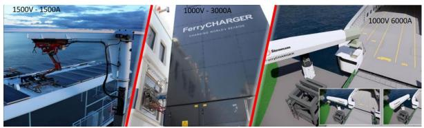
Figure 4: Typical ACD systems with from left to right: PANTO type, Tower type and BOW type
